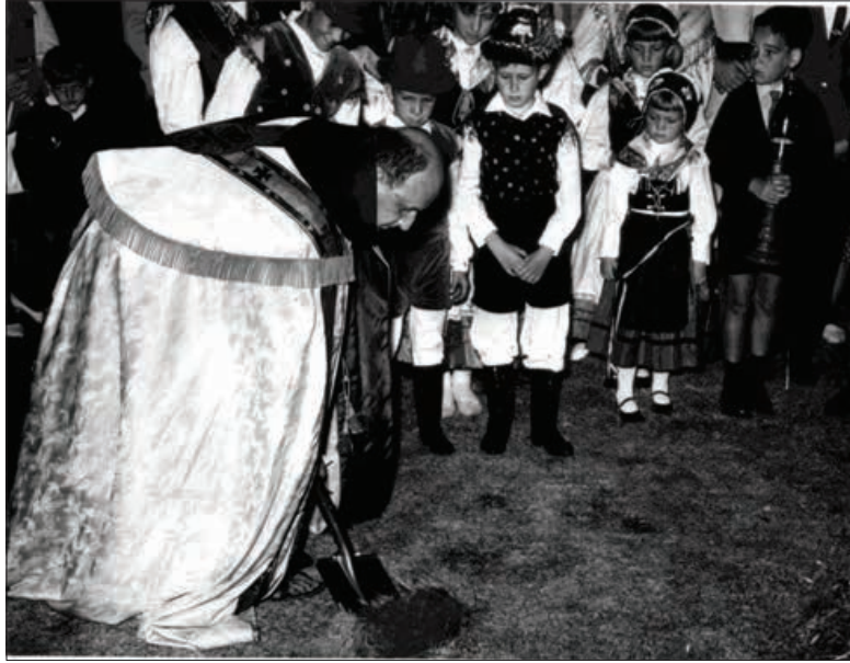
On Sunday March 7th 1965 we planted the first shovel and blessed the building site.
